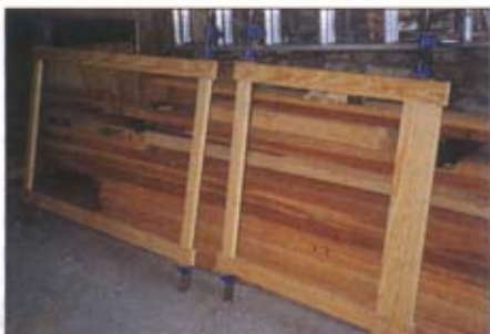
The upper and lower frames glued and cramped
