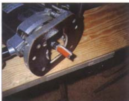
I used a pattern cutter to trim the top and bottom of the doors square and to size. The bearing runs against a straight batten cramped to the door
