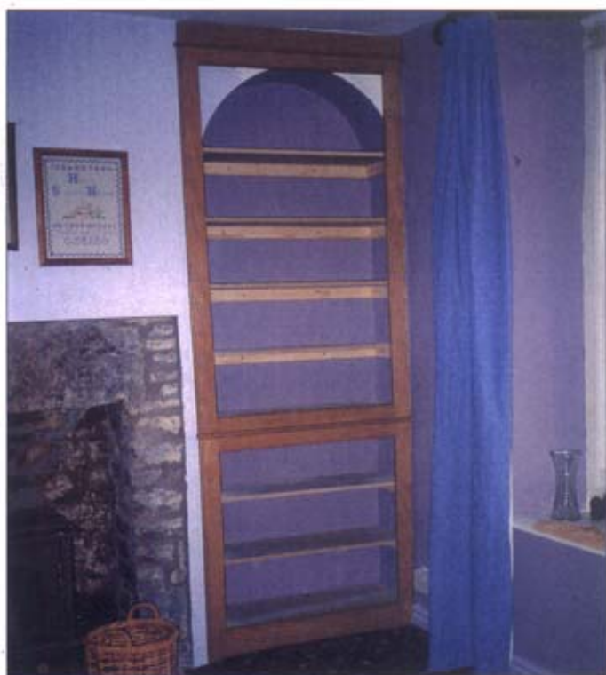
The frames fixed in position, ready for the doors to be fitted
