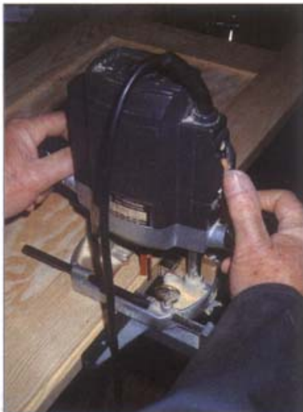
Cutting the rebate on the meeting stiles of the doors
