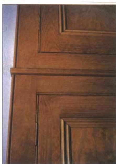
A hinges are set into the doors only so that they follow the line of the bead
